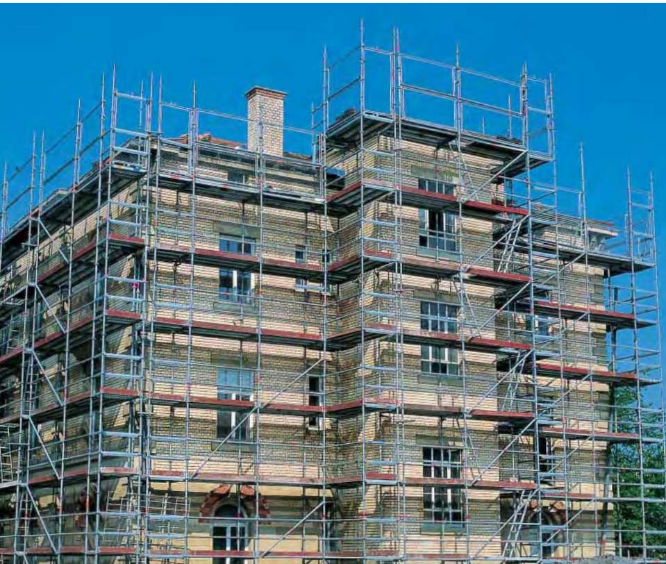
Facade scaffolding for heavily structured facades
