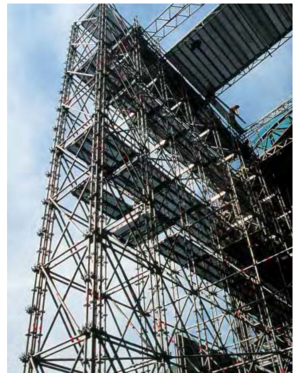
Falsework in industrial construction, bridge-building and solid construction
